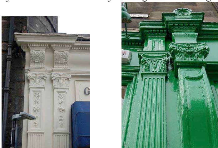
Consoles and pilasters
