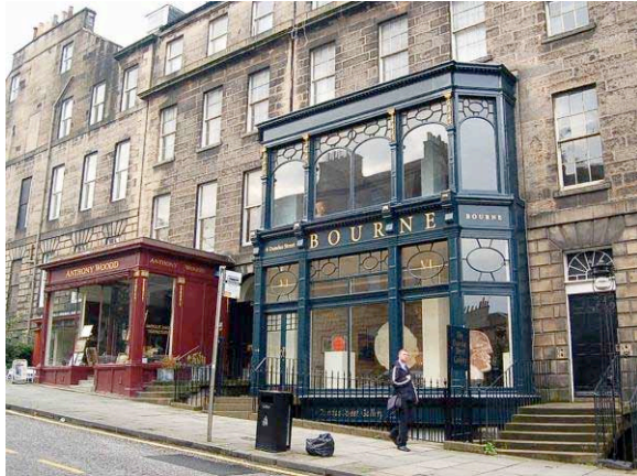
Shops built over basements, Edinburgh
