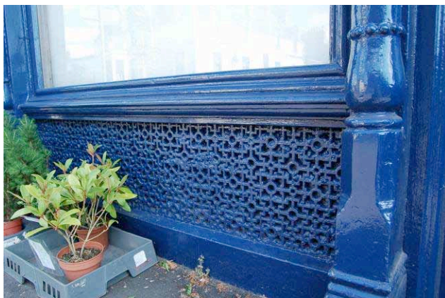
Stallriser using decorative fretwork
