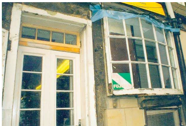
Shopfront under repair
