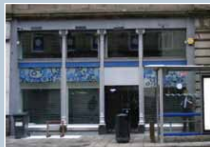
One of the cast-iron shopfronts that came to light during recent refurbishment of Dundee's Improvement Act streets.
