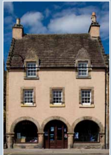
Braco's Banking House (1694), High Street, Elgin. In the late 17th century a number of Scottish burghs adopted a continental model of arcades at the ground floor to house shops.
