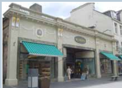
Replacement fabric attached to the traditional awning mechanisms at McEwens, St John Street, Perth.
