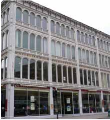
Gardner's Warehouse, Jamaica Street, Glasgow. Now in use as a bar, this pioneering iron-framed building was constructed as a retail warehouse in 1855-6 for A Gardner & Son, cabinet makers and upholsterers. The original lettering was kept at first floor, and new lettering in a similar style fitted to match the new name at the ground floor.
