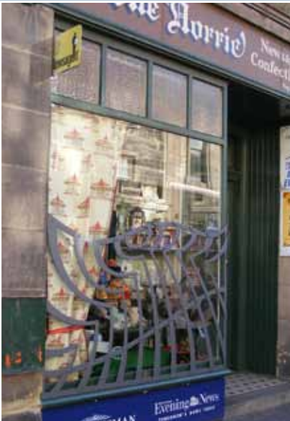
These modern removable external grilles by an artistic blacksmith were put into shops in place of less attractive fixed mesh as part of the Bo'ness Townscape Heritage Initiative.
