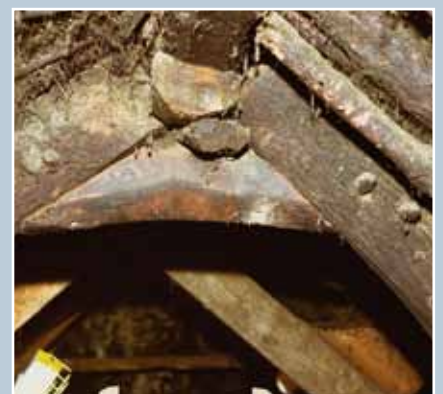
Hand-hewn roofing timbers pegged together in a late 18th- to early 19th-century cottage. Pitlochry, Perth & Kinross.
