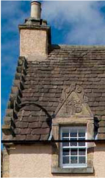
Graded stone slates, laid in diminishing courses from the bottom to the top of the roof. Associated features include crowstepped gables, a corniced chimney and a decorative dormerhead dated 1694. Elgin, Moray. © N Haynes.
