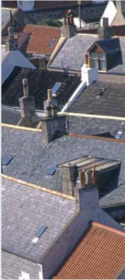
The Seatown at Cullen, Moray, showing a wide range of slated and pantiled roofs. The Scots slate here is darker and smaller than the more regular blue Welsh slate. Pantiles were commonly used in Eastern Scotland where cheaper and well-ventilated roofs were needed, but slate was preferred on most houses.
