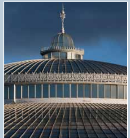
Glazed roof at the Botanic Gardens, Glasgow City. © N Haynes.
