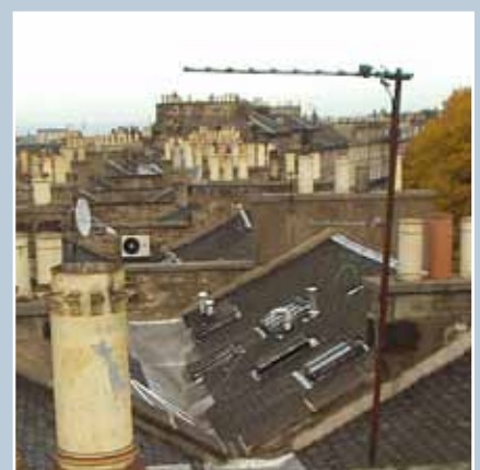
Aerials, vents, rooflights, satellite dishes and air conditioning units located in roof valleys to minimise impact.
