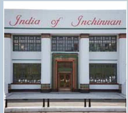
India of Inchinnan tyre factory restored, extended and converted to offices in 2002.
