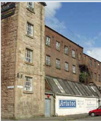
Falfield Mill, an 1818 cotton mill in Glasgow was one of two listed buildings demolished on the route of the new M74 extension, an infrastructure project of national significance.
