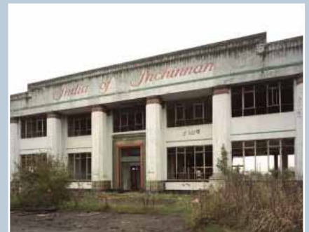
The 1929 Art Deco India of Inchinnan tyre factory, Renfrewshire, shown derelict and threatened with demolition in a photograph taken in 1992. © Crown copyright: RCAHMS. Licensor www.rcahms.gov.uk .
