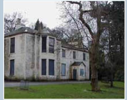
Linn House, Glasgow. A demolition application was submitted with no marketing evidence, but later withdrawn when restoring purchasers came forward.
