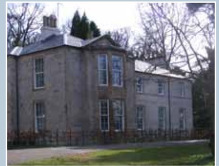
Linn House, Glasgow, repaired and extended (photo 2009).
