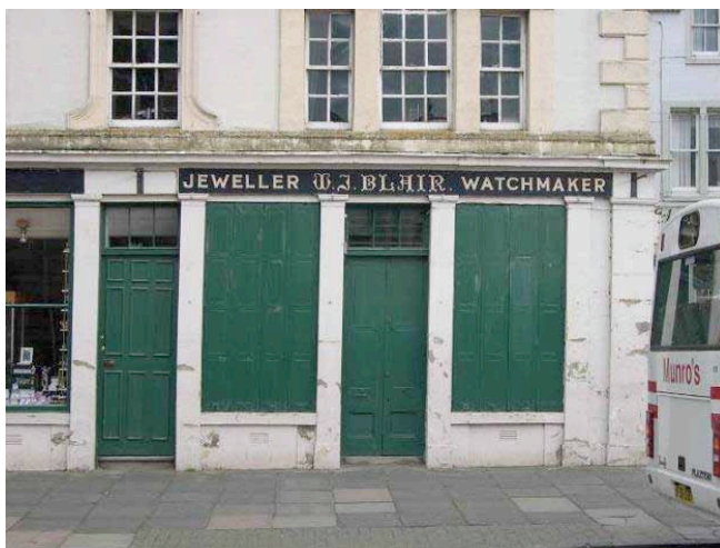
19 th century shopfront with original shutters
