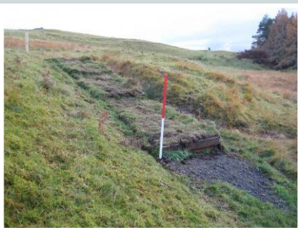
Small areas of earthwork repair can often halt the erosion on a scheduled monument.
