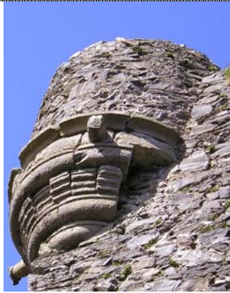
Fig. 112 Castle Tioram: specimen angle turret
