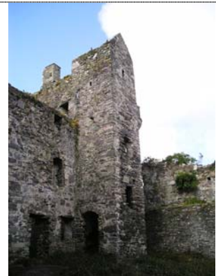
Fig. 114 Castle Tioram: stair turret, south courtyard range from ...
