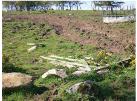
The remains of a pre-improvement farmstead near Mintlaw, Aberdeenshire overlies an earlier settlement and field system some 4,500 years old. The use of farm vehicles and erosion from cattle, particularly around the feeder, has caused damage to the site.
