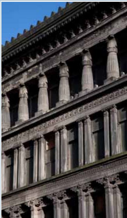
Egyptian Halls by Alexander 'Greek' Thomson in Union Street, Glasgow, 1871. Thomson's Graeco-Egyptian design emphasised the solid monumentality of the masonry against the void of the window openings. He used large sheets of plate glass and minimal dark-painted frames to achieve this effect. © N Haynes.
