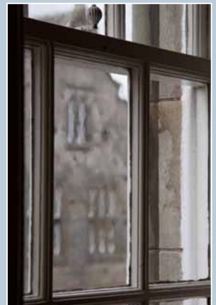
Detail of a timber sash and case window of circa 1890 showing the profile of the astragals, the irregularities of the glass, and a decorative sash fastener. © N Haynes.
