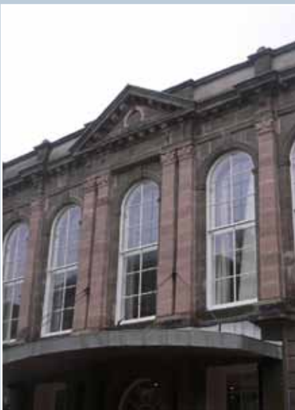
Webster Theatre, Arbroath. Large clear sheets of internal secondary glazing were installed here during recent refurbishment.
