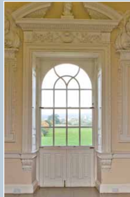
This original window/door of the 1730s at Chatelherault, Hamilton, illustrates the principle of converting a window to a door. In order to maintain the consistency of architectural treatment in the room, the upper part of the door is treated as a window, and the lower section is solid.
