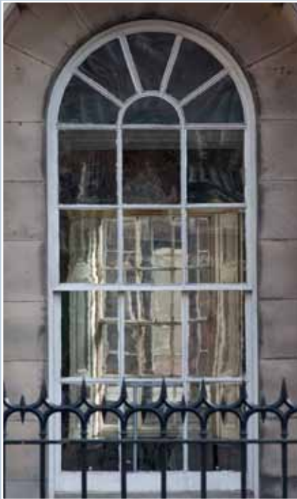
A round-headed cylinder glass sash and case window with slim 'astragals', or glazing bars of circa 1810, Signet Library, Parliament Square, Edinburgh. Irregularities in the glass provide the variety and individuality of the reflective pattern. © N Haynes.
