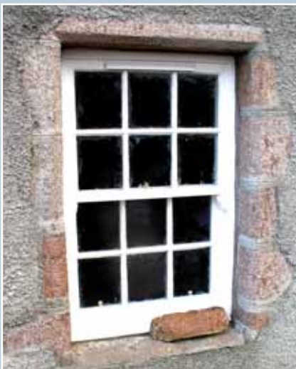
A new single-glazed window detailed to match the previous window, except that horns have been added to the top sash, not necessary where the astragals give rigidity, and a 'permavent' has been added. See page 7 for an alternative ventilation method.
