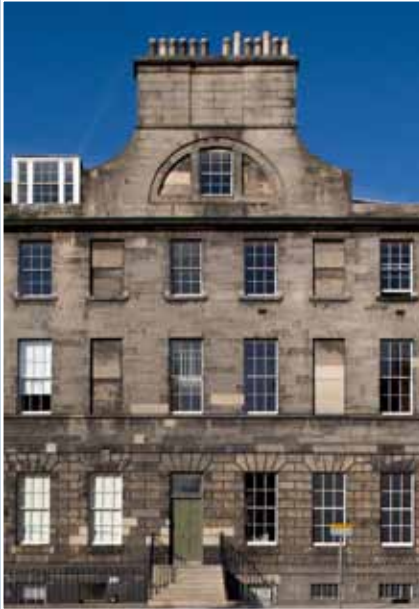
South Charlotte Street, Edinburgh. The blind openings are detailed with sills and a 'meeting rail' to maintain the symmetry of the architectural elevation. The chimney flues pass behind the blind windows. © N Haynes.
