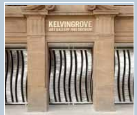
New wide openings were created at the rear of Kelvingrove Art Gallery in Glasgow to provide level access to the building. The scheme used the existing architectural stone framework to set off new high-quality gates sculpted in stainless steel.
