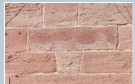
High Street, Arbroath. Rich pink-red sandstone, typical of parts of Angus. Here the stone is laid in regular courses. © N Haynes.
