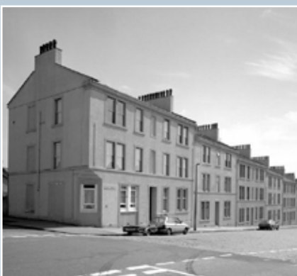
Mass concrete tenements in Dundee, cast in-situ in 1874–5 by the Concrete Building Company for the Working Men's House Building Association. The buildings were renovated and a buff render applied in 1982–4. © Crown copyright: RCAHMS. Licensor www.rcahms.gov.uk .
