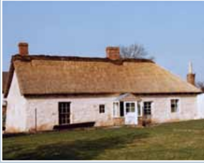
The mid 18th-century Old Schoolhouse at Cottown, Perth & Kinross. The uneven character of the wall surface is derived from the local materials used in its straw-bonded mudwalls. The colour reflects the use of local clay as a pigment in the modern coating of lime harl and limewash applied during repairs by the National Trust for Scotland. The different window sizes reflect the internal hierarchy of rooms. © N Haynes.
