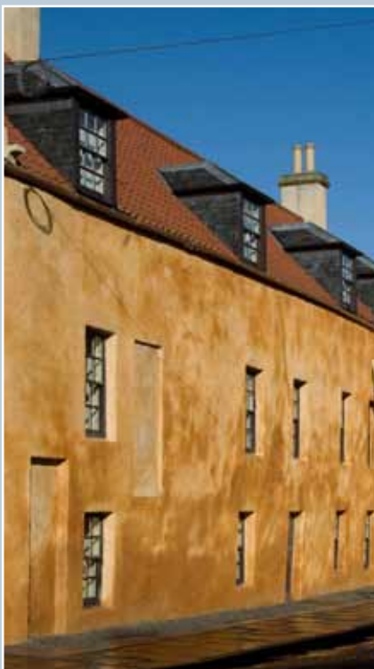
Dymock's Buildings (late 17th century), Bo'ness, was restored by the National Trust for Scotland in 2004. A cement render was removed, the archaeology of the wall recorded, and then a lime harl and limewash were applied. Evidence of former openings remains visible. © N Haynes.
