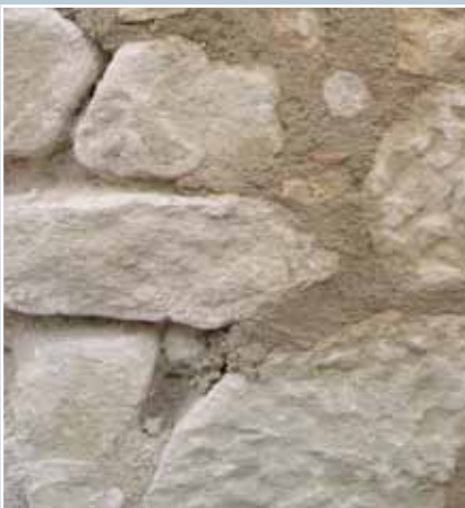
Modern lime mortar pointing, Scottish Lime Centre, Charlestown, Fife. The use of lime allows the wall to 'breathe'. Traditionally, most rubble walls had lime slastered, or buttered, over the joint to achieve a fairly smooth finish that would erode with time. Where pointing does not alter the character of a listed building it would not normally require consent.
