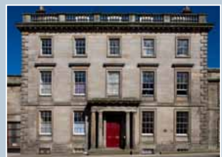
Central block of the former Fife Arms Hotel, Banff, 1843–45. The classical design places emphasis on the symmetry, proportions and detailing of the walls and reflects the functional hierarchy of the interior. Corniced windows indicate the principal rooms on the first floor; smaller windows relate to private or subsidiary rooms. The design maximises the architectural impact of the walls by hiding the shallow pitched roof behind a parapet. © N Haynes.
