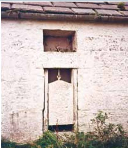
A cheese press built into the wall of a farm cottage at Reay, Highland. Although the press is no longer used, it provides insight into the type of farming of the area and old methods of cheese production.
