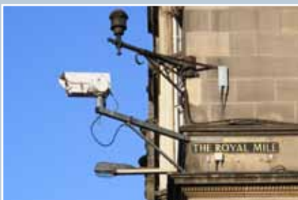
Here the corner profile of the building is broken by the brackets for a security camera, an old lamp, and modern street lamp.
