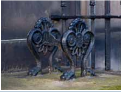
An elaborate cast-iron bootscraper at the entrance to a house in Randolph Crescent (1829), Edinburgh. Such fixtures were common in the early 19th century when road surfaces were generally muddy. © N Haynes.
