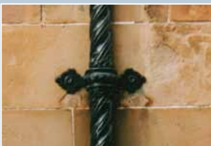
A later 19th-century cast-iron 'barleysugar' downpipe and decorative bracket in Rothesay, Isle of Bute. © N Haynes.
