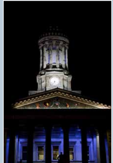
Gallery of Modern Art, Glasgow. The floodlights are positioned behind a cornice and on the roof, therefore making little impact in daylight but providing atmospheric lighting after dark. © N Haynes.
