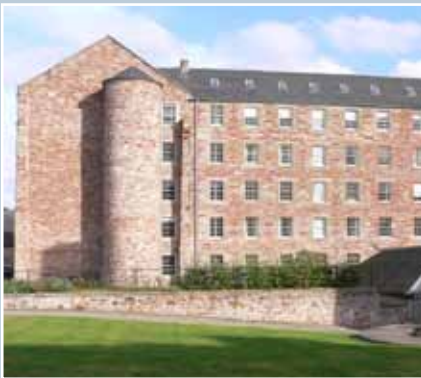
Complementary: Stanley Mills, Perth and Kinross. A new lift tower was added to East Mill that echoes a semicircular stair tower on nearby Mid Mill. The location had been scarred by an earlier lift and rudimentary toilets. A glass strip separates the new-build from the historic masonry.
