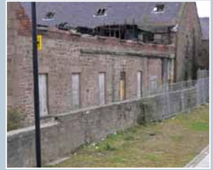
Former Arctic Tannery and Harbour Workshops, Dundee. A fire destroyed the upper part that had originally been of timber louvres to cure sealskin hides, replaced in brick. The development of housing (below) echoes in a new form the timber and brick previously used here.
