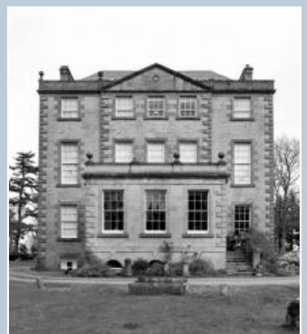
A house of 1776 in Morayshire before the removal of an 1870 porch. © Crown copyright: RCAHMS. Licensor www.rcahms.gov.uk .
