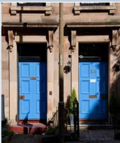
The door on the left is redundant following the internal amalgamation of two villas, but retained in place to maintain the character of the building. © N Haynes.
