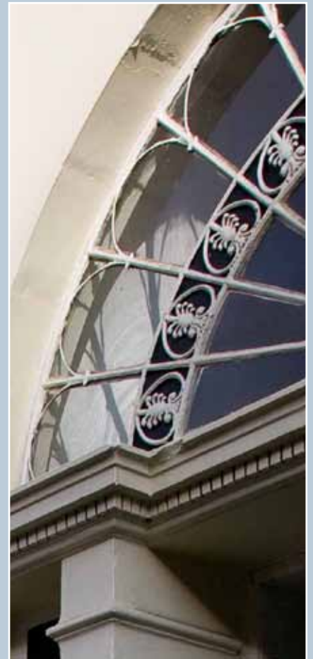
Detail of a delicate cast-iron fanlight dating from the 1790s in Edinburgh. © N Haynes.
