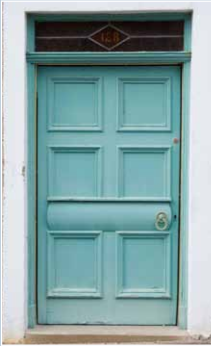
A timber panelled door in the Seatown at Cullen, Moray. The detailing of this door is typical of the high-quality joinery of the area. Draught-proof strips have been applied around the door. © N Haynes.
