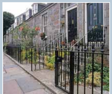
Albert Terrace, Aberdeen. Designed by the architect Archibald Simpson in about 1840, the paired doorways form part of a consistent architectural pattern throughout the terrace of houses. Additional features include the steps and decorative iron railings.
