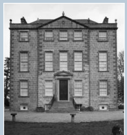
The same house with the porch removed and the principal elevation carefully restored to its 18th-century form on the basis of documentary research. © Crown copyright: RCAHMS. Licensor www.rcahms.gov.uk .
