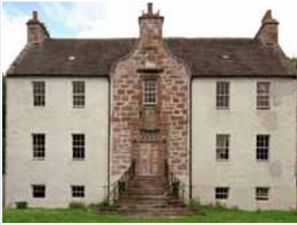
The doorway, with its stair, stone surround, decorative fanlight and heraldic panel, is the principal feature of this symmetrically designed Ross-shire house of 1760. © Crown copyright: RCAHMS. Licensor www.rcahms.gov.uk .
