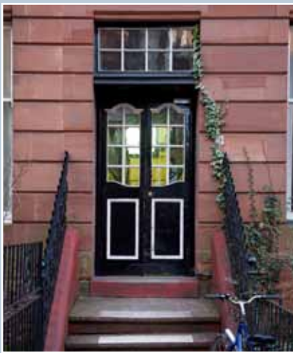
Glazed upper panels form an original feature of this Glasgow tenement door. © N Haynes.
