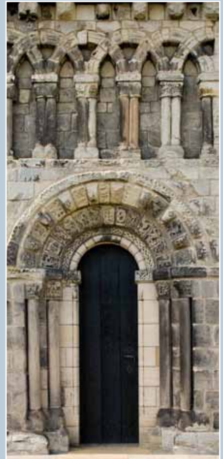
The exceptional 12th-century Romanesque doorway at Dalmeny Parish Kirk. Like many early church doorways, it is decorated with symbolic carvings. The door and inner stone frame are 20th-century replacements. © N Haynes.
