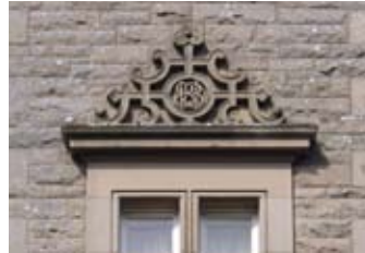
Woodnorton, tower detail
