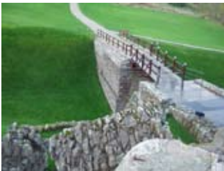
View across drawbridge
