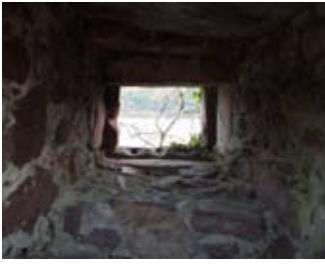
Window in store room
