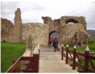
Drawbridge and gatehouse
