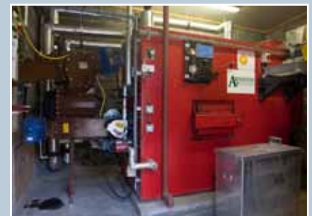
Above and below: an ancillary building at Arniston House, Midlothian, was converted to a boiler room and fuel storage for a 460kW wood-chip biomass system. The new flue is detailed to match the existing chimneys. Wood-chip fuel is sourced locally and fed into the store using a moveable agricultural conveyor. © N Haynes.
