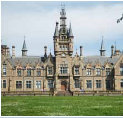
Morgan Academy, Dundee, where micro-renewables have been incorporated sensitively. Ground- and air-source heat pumps are powered by photovoltaic panels located in the hidden valleys of the roof.
