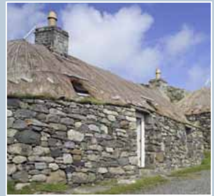
Blackhouses at Garrannan, Isle of Lewis, refurbished for self-catering holiday and hostel accommodation. Three ground-source pumps totalling 51kW output were installed at one central location to service seven cottages. The effect on the character of the buildings is minimal. © Crown copyright: RCAHMS. Licensor www.rcahms.gov.uk .
