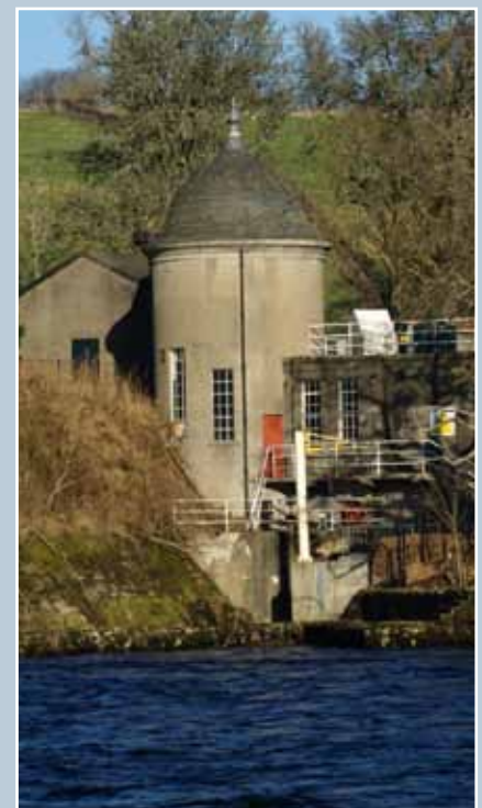
1921 turbine house, Stanley Mills, Perth & Kinross, recently refurbished as part of a new hydro-electricity scheme to supply power to the grid. At 840 kilowatts the scheme is significantly larger than a standard micro-renewable development, but it demonstrates the potential for reuse of an existing historic hydro site.
