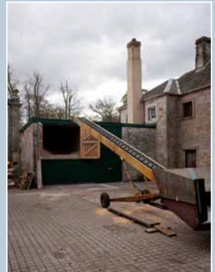
Above and below: an ancillary building at Arniston House, Midlothian, was converted to a boiler room and fuel storage for a 460kW wood-chip biomass system. The new flue is detailed to match the existing chimneys. Wood-chip fuel is sourced locally and fed into the store using a moveable agricultural conveyor. © N Haynes.
