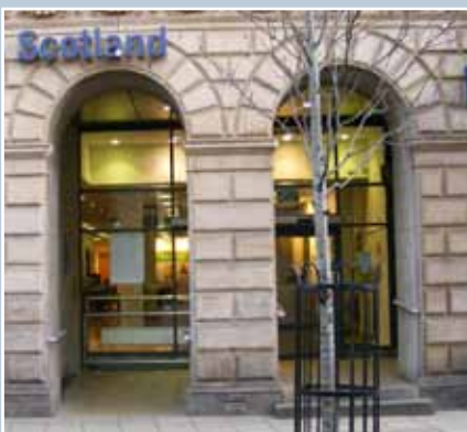
Kirkcaldy, Fife. Ramped and stepped access was achieved in this busy pedestrian street by removing the original door and a window to create an internal lobby. Equality of access was achieved and the principal feature of the building's ground floor, the arcade of round-headed arches, was maintained.
