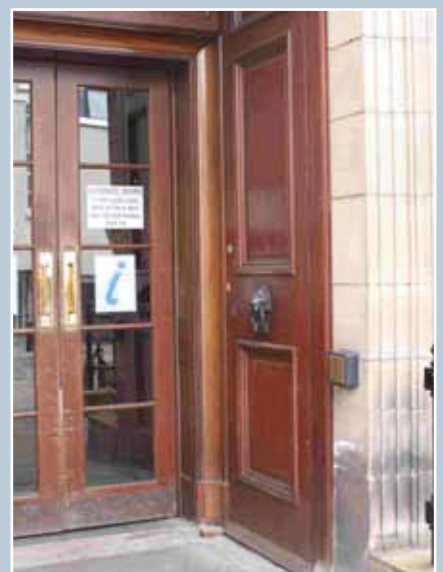
The door into Linlithgow's County Buildings opens automatically, and also has a manually operated push pad. © West Lothian Council.
