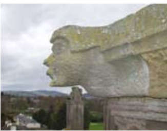
Waterspout on roof
