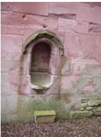
Wash place at foot of night stair
