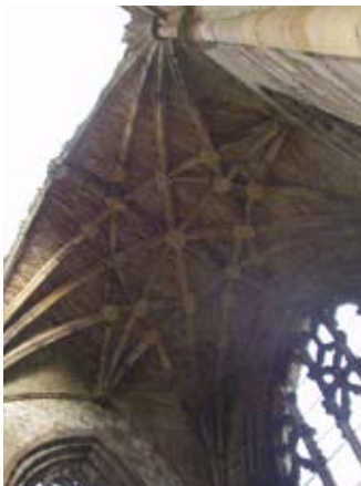
Vaulting in Presbytery
