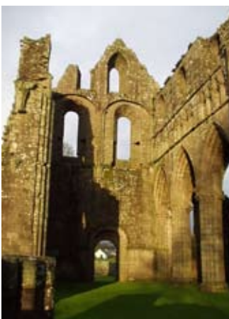
View north at crossing
