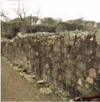
North wall of cloister
