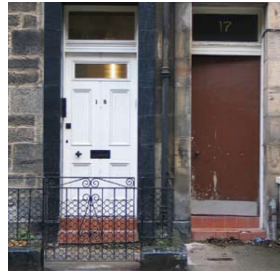
The difference between retaining a traditional door and a poor quality replacement.
