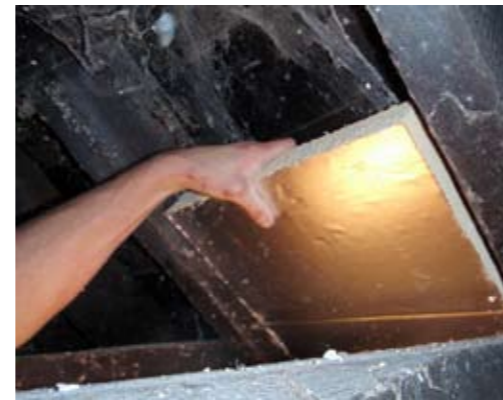
Fig 2. Insulation board can be cut to fit between rafters
