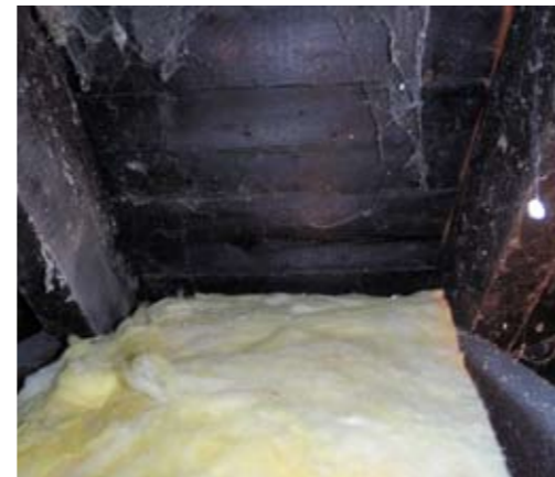
Fig 3. Mineral wool insulation can also be laid between rafters and joists, but with care not to inhibit air movement.
