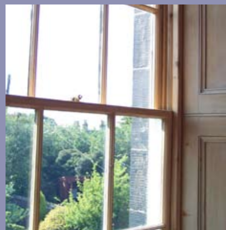
Fig 10. Existing sashes re-glazed with DG units.
