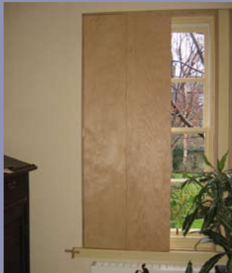
Fig 9. Modern shutters fitted to a traditional window. Jonathan Gotelee Architects
