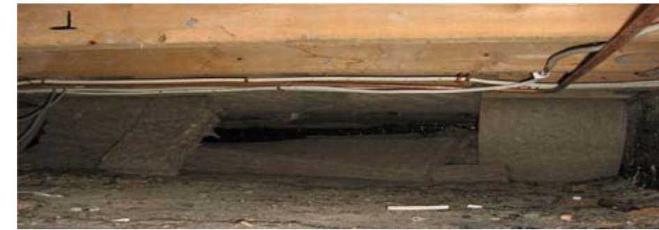
Fig 4. Fitting of natural insulation underneath a timber floor
