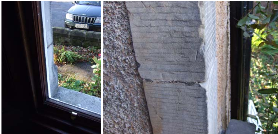
Figure 10 – window and sandstone wall of detached house (variant 3)
