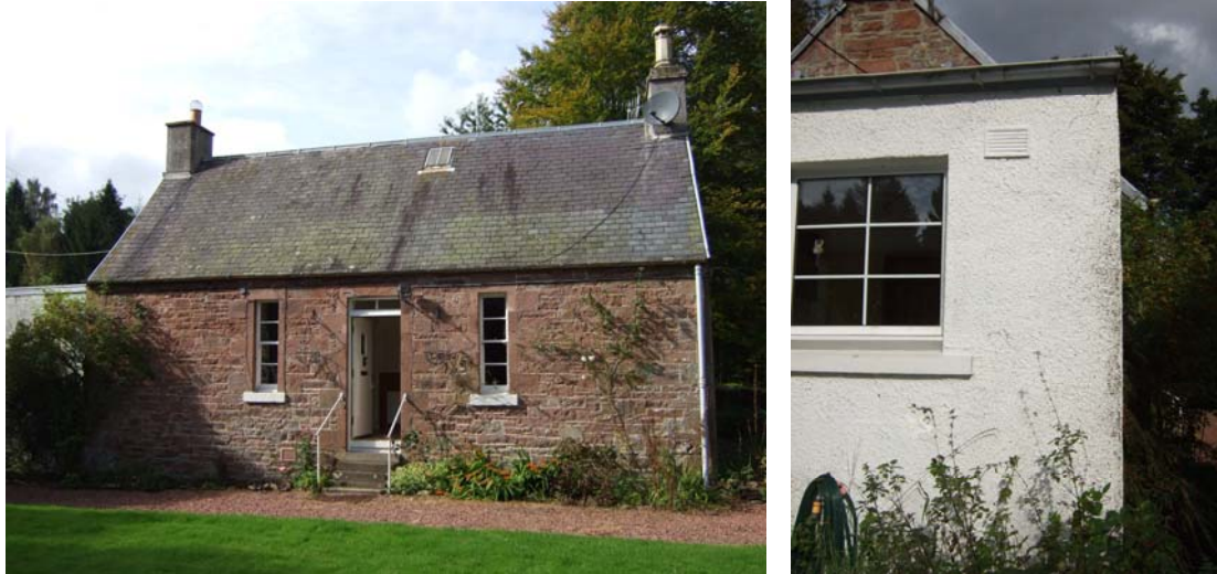
Figure 5 – Cottage (with extension) used for variant 2
