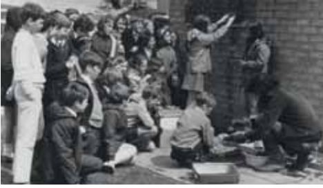
David Harding supervises as children place their tiles in Huntly Drive (1971)
