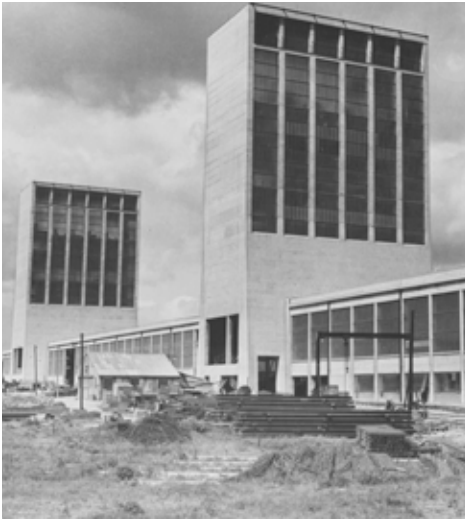
Construction of the Rothes Colliery (1956)
