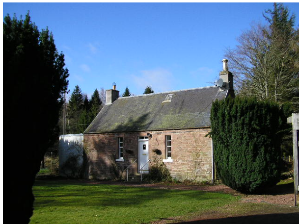
Figure 14: Weens Cottage, Borders Red sandstone & brick Four measurement locations Wall thickness: 400mm External face: rubble (x3) and cement (x1) Internal face: hard plastered
