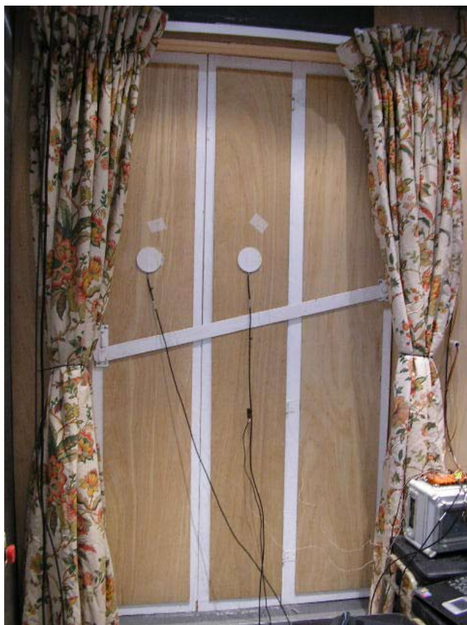
Figure 6: Insulated shutters installed
