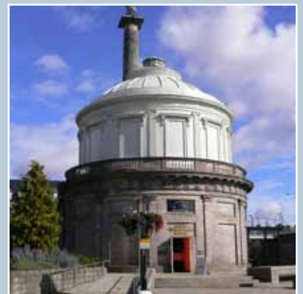
Perth Water Works, now converted for use as the Fergusson Gallery, has a cast-iron cistern made in 1832 that has recently been refurbished.
