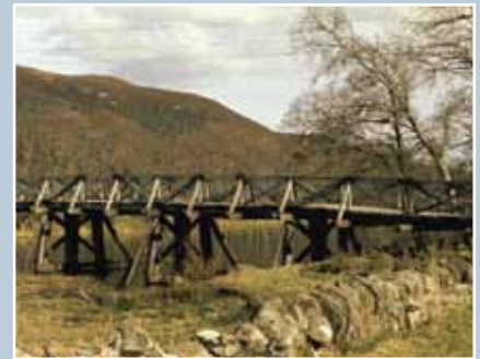
This bridge at Garve, Highland, is one of only four of its type to survive. Built during the late 19th century, the bridge is of timber trestle construction, and consists of eight spans, with six main truss spans. © Crown copyright: RCAHMS. Licensor www.rcahms.gov.uk .
