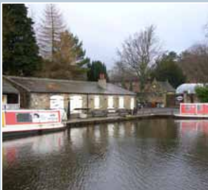
A basin on the Union Canal at Linlithgow, West Lothian, which following the completion of the Millennium link, is seeing increasing leisure uses alongside and on the canal. Most maintenance work, such as to the puddle lining of a canal, is covered by class consents. © N Haynes
