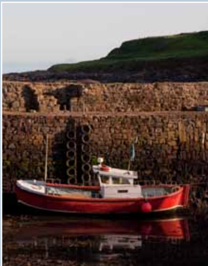
Vertical coursed masonry at Pittenweem Harbour, Fife. © N Haynes.
