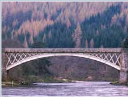
Carron Bridge, Moray, 1863: a railway bridge that is now a road bridge. An application to build a new steel arched bridge, and fix the outer cast-iron ribs to it, was withdrawn after it was found by calculation at a public inquiry to be unnecessary. The cross spandrels read through from side to side, so facadism was not going to work visually.
