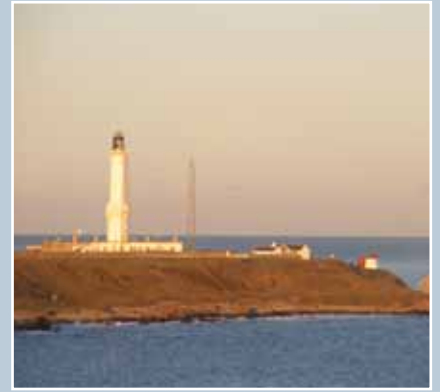
Girdleness lighthouse, Aberdeen, 1833, has typical keepers' houses, flat-roofed to emphasise the height of the tower, a compressor house and foghorn. A radio mast makes it a key part of the UK Global Positioning System (DGPS) and is not out of place.
