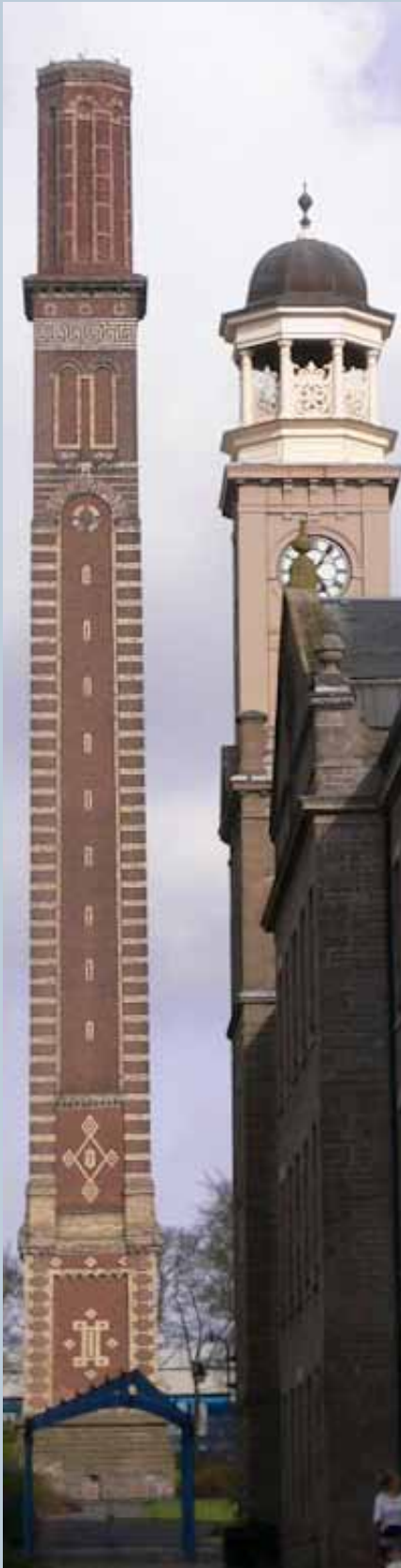
Cox's Stack: a 90-metre-high sentinel over Camperdown Works, Dundee, 1865, is the focal point for a mixed use urban regeneration project. Red and white polychrome brick was popular in industrial buildings from 1860 to 1880. A proposal to fit a large dot matrix sign to the upper stage was refused following a public local inquiry.
