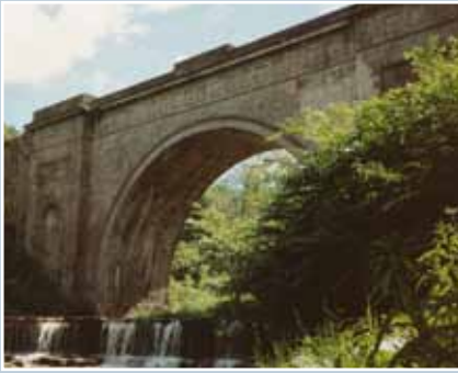
Montagu Bridge, Dalkeith, Midlothian, by Robert Adam, 1791. For reasons of picturesque variety Adam constructed a small cauld, or weir, downstream. Water tumbles over the cauld and the noise is amplified by the echo of the underside of the bridge; upstream the other side of the bridge is reflected in the calm waters held back by the cauld. The noise and reflective qualities of the water contribute to the setting of the bridge.
