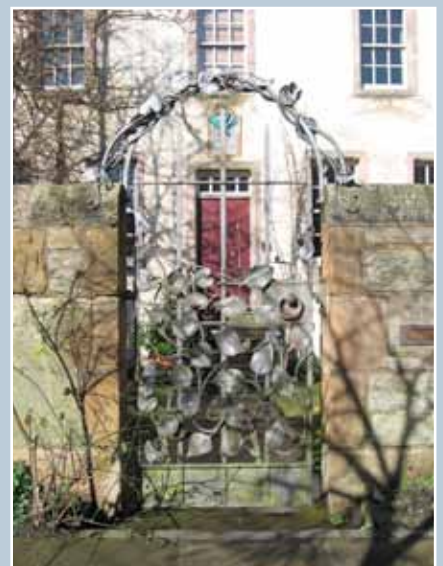
St Leonard's, Edinburgh. An early 18th-century house restored in 1982 with contemporary ironwork to garden gate and entrance railings.
