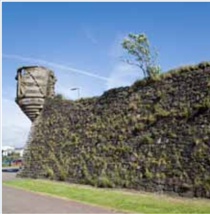
Part of the Citadel wall in Ayr, designed by the military engineer, Hans Ewald Tessin, in 1652 to protect Oliver Cromwell's garrison in the town. The corner turret is a 19th-century folly. The surviving walls of this large military complex are now in multiple ownership. © N Haynes.
