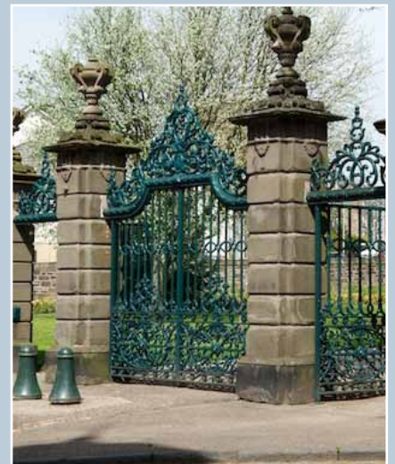
Baxter Park, Dundee. The cast-iron gatepiers and cresting of 1863 survived, but the gates were missing until they were replaced as part of the restoration of the park in 2007.
