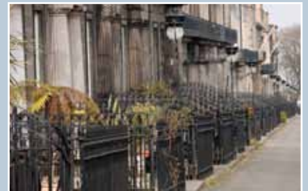
A long complete stretch of iron railings and lamps at Regent Terrace, Edinburgh, part of the development planned by William Henry Playfair in 1825 and built 1826–33. © N Haynes.
