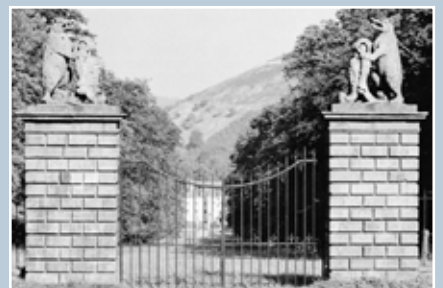
The 'Bear Gates', Traquair House, Scottish Borders, constructed in 1737–8. Part of their historical and associative interest is a legend that relates the gates were closed behind Bonnie Prince Charlie in 1745 and have not been opened since. © Crown copyright: RCAHMS. Licensor www.rcahms.gov.uk .
