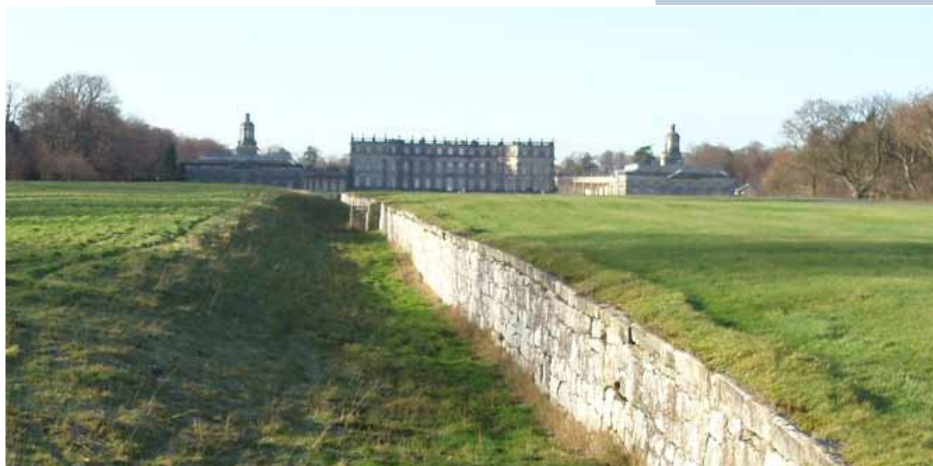
Hopetoun House, West Lothian, viewed from beyond the haha. The sunken wall and ditch allowed unobstructed views from the house, but kept livestock out of the garden.
