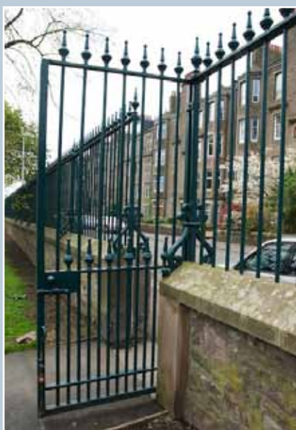
Railings reinstated in 2006 define the edge of Baxter Park, Dundee, and are key to its regeneration and good management. The patterns were deduced from a short surviving section.
