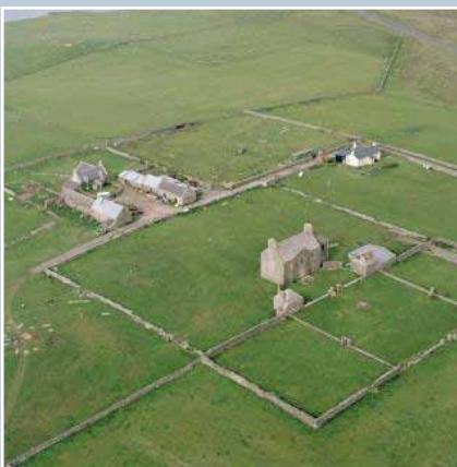
Like many 18th- and 19th-century buildings in Shetland, Belmont House (1777), Unst, stands at the centre of an extended formal arrangement of field boundaries. This aerial view was taken in 2005 before the recent restoration of the house. © Crown copyright: RCAHMS. Licensor www.rcahms.gov.uk .
