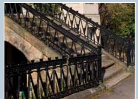
Circa 1865 cast-iron railings at a tenement in Sanda Street, Glasgow. © N Haynes.
