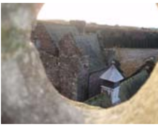
View to kitchen tower from rooftop
