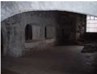
Serving hatches in the kitchen
