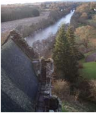
View west from rooftop
