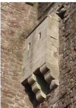
Latrine on west wall
