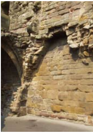
Remains of Fireplace in kitchen
