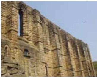
Refectory from kitchen
